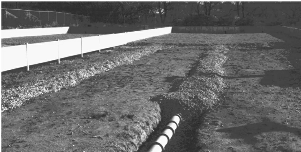
FIGURE 26.16 Conventional sand drying bed with tile underdrain system, shown here during
