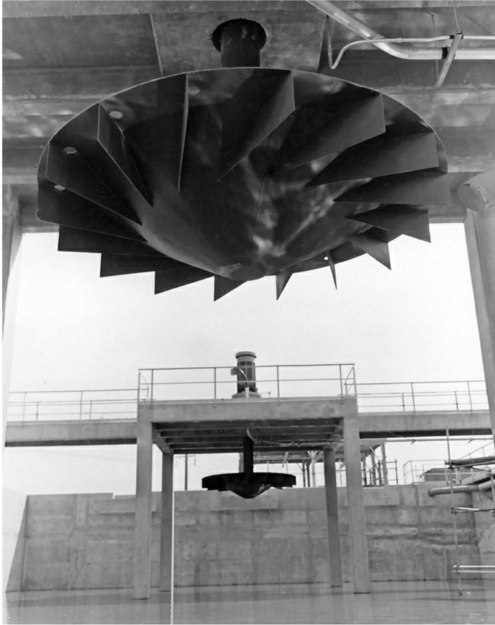
FIGURE 29.10 Details of construction of a fixed-position surface aerator, shaped to produce high-volume pumping and air entrainment. ( Courtesy of Infilco Degremont Inc. )
