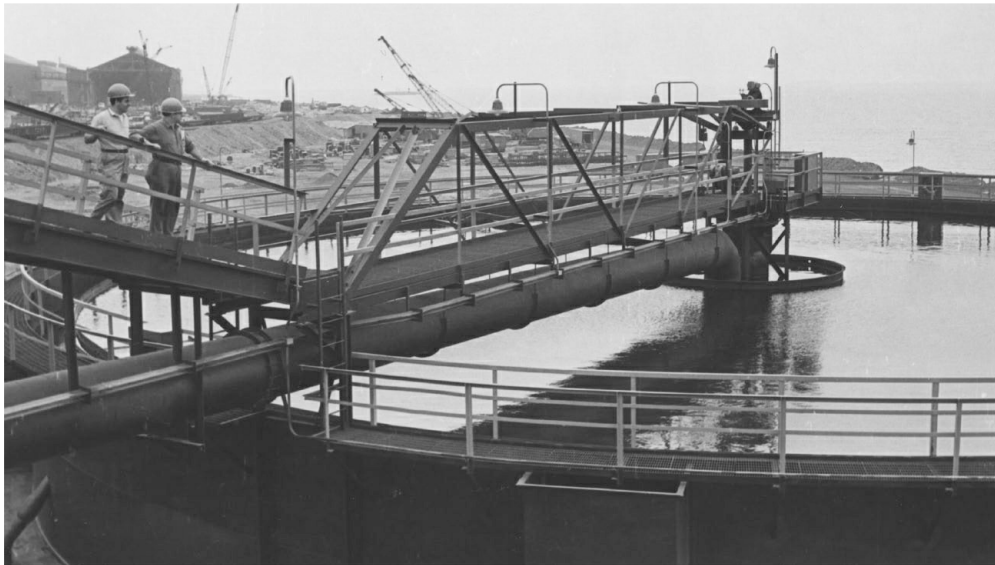
FIGURE 38.3 Clarifier-thickener used to treat blast furnace gas scrubber water and to recover solids. (Courtesy of Inland Steel Company.)
